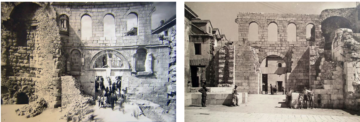
Fig. 4: East-Gate. Left (a): Opening of the Gate during the conservation works, 1945 (CD/MC/Split). Right (b): After the Conservation works, 1945 (CD/MC/Split).
