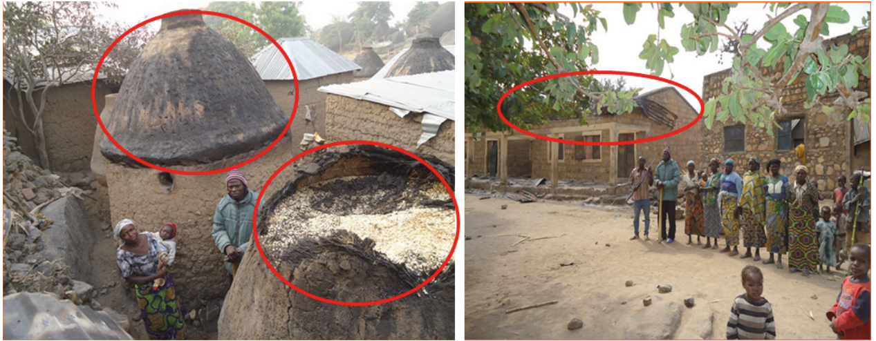
Fig. 6: Building burnt by the Insurgents (Photos: Stefan Kiehas & Simon Zira).
