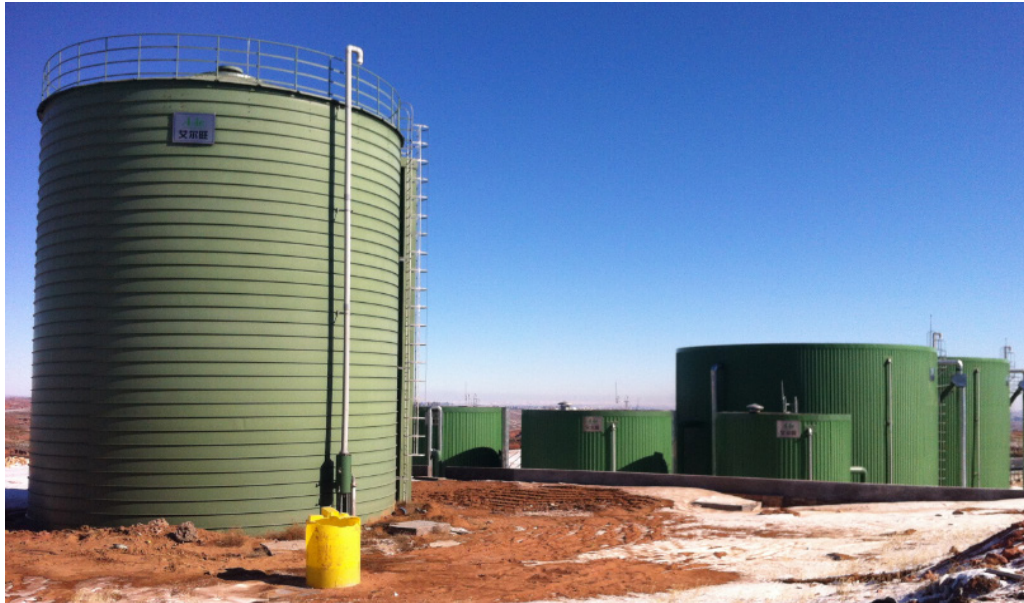
Figure 1-6: Kangbashi Biogas Plant, Erdos, China, 2012
