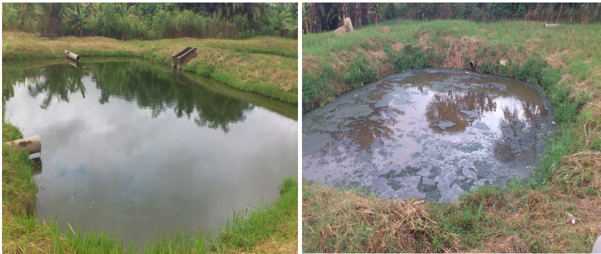
Figure 5: Stabilization ponds for the Ahinsan and Chirapatre communities (Field photograph, 2014)
