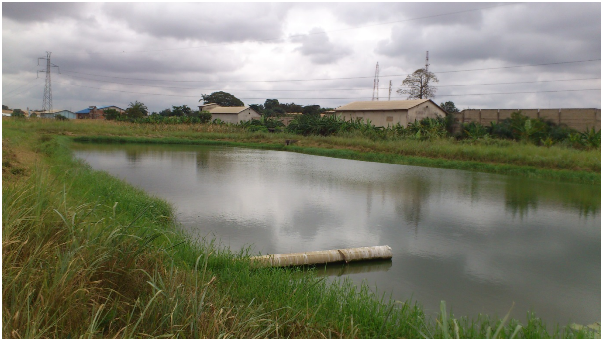
Figure 4: Asafo waste stabilization pond (Field photograph, 2014)
