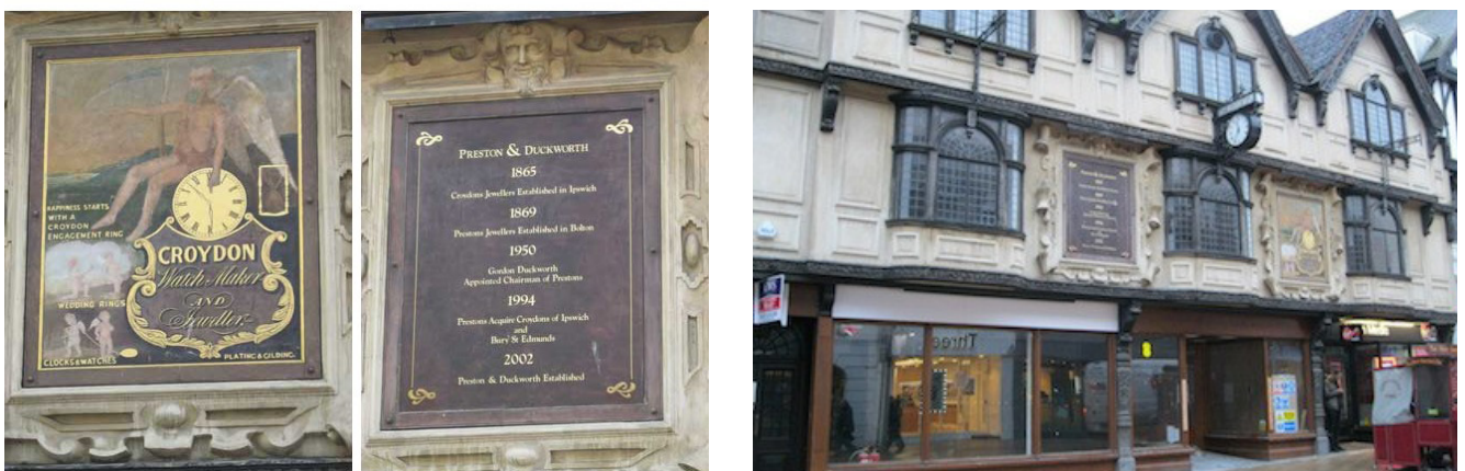
Abb.2: Vorderfront und Fassade des Croydon Buildings in Ipswich. © Copyright Borin Van Loon (www.ipswich-lettering.co.uk) (Quelle: http://www.ipswich-lettering.co.uk/tavernstreet.html )
