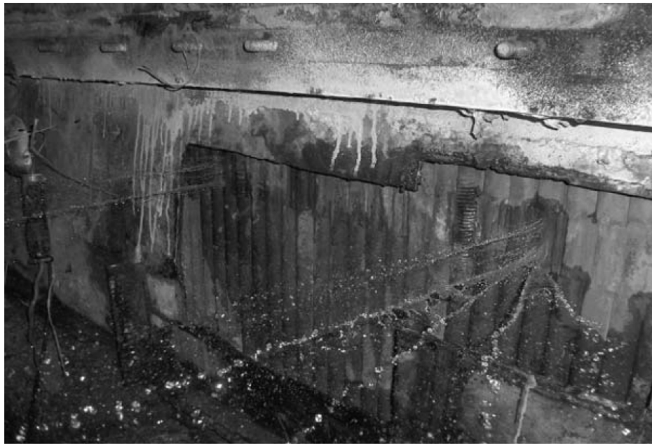
(a) Leakage tubes caused by thermal transients, [7]
