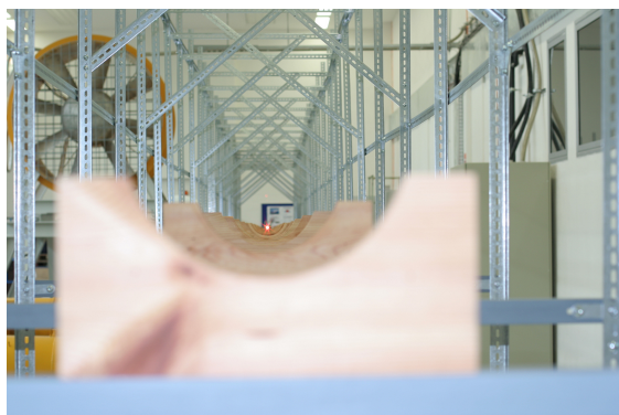
(a) Sub-construction of the CoLaPipe with a laser point at the end marking the position of the blower unit. The theodolite and the surveying level are used to set up the sub-construction as well as to establish the connection to the blower unit.
