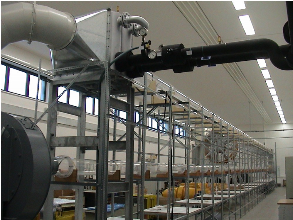
Figure 4.13: Rear view of the test facility from the blower and cooling unit with the actual test section and the return line.
