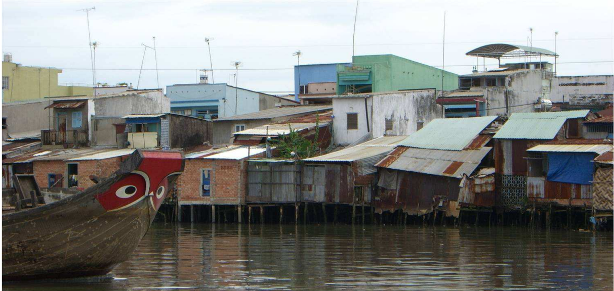
Fig. 2-2: Waterside Settlement, District 8, HCMC (Photo: Schinkel 2008)
