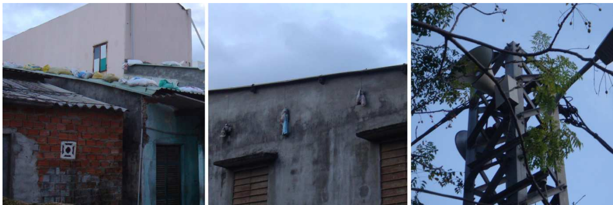
Fig. 2-17: Response Measures Applied prior to the CBA Transfer Project (Photos: Schinkel 2013)
