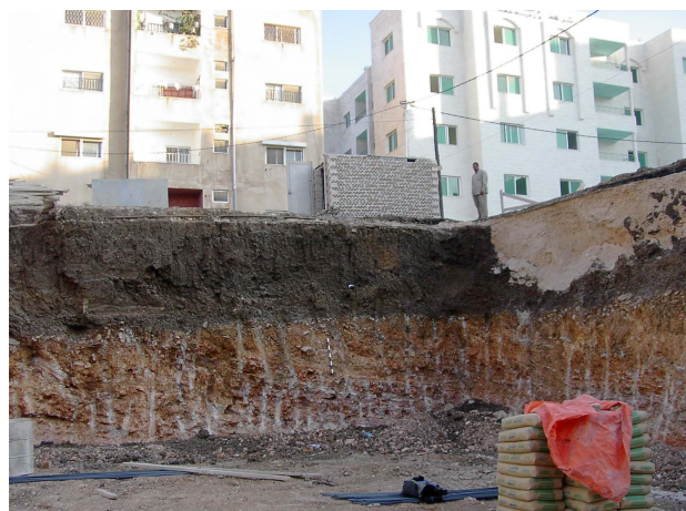
Figure 23: Sampling the building pit in Irbid.
