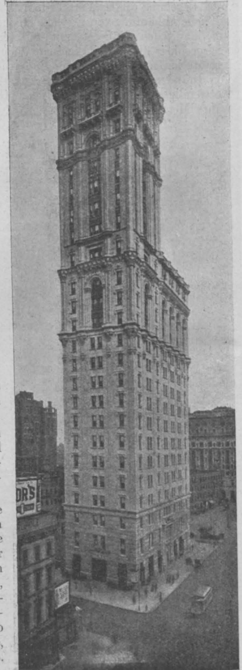
Abb. 17. Das Times Building in New York.
