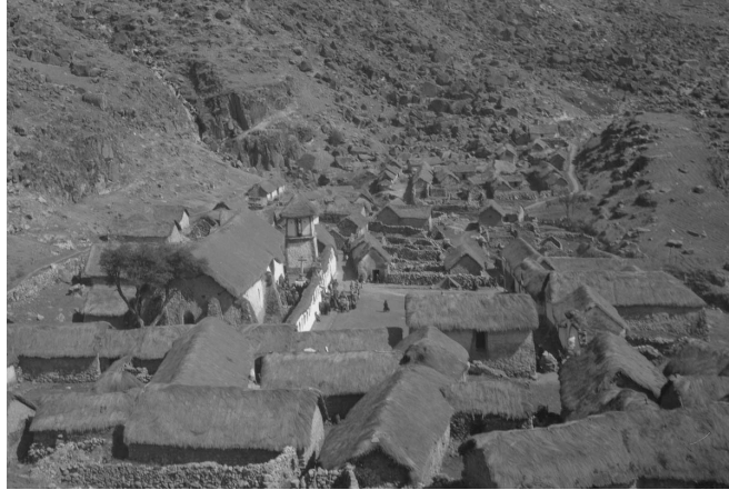
Figure 23: Vernacular architecture from the Andean region. Stone foundations, adobe walls and ichu roofs, circa 1930. ©Martin Chambi
