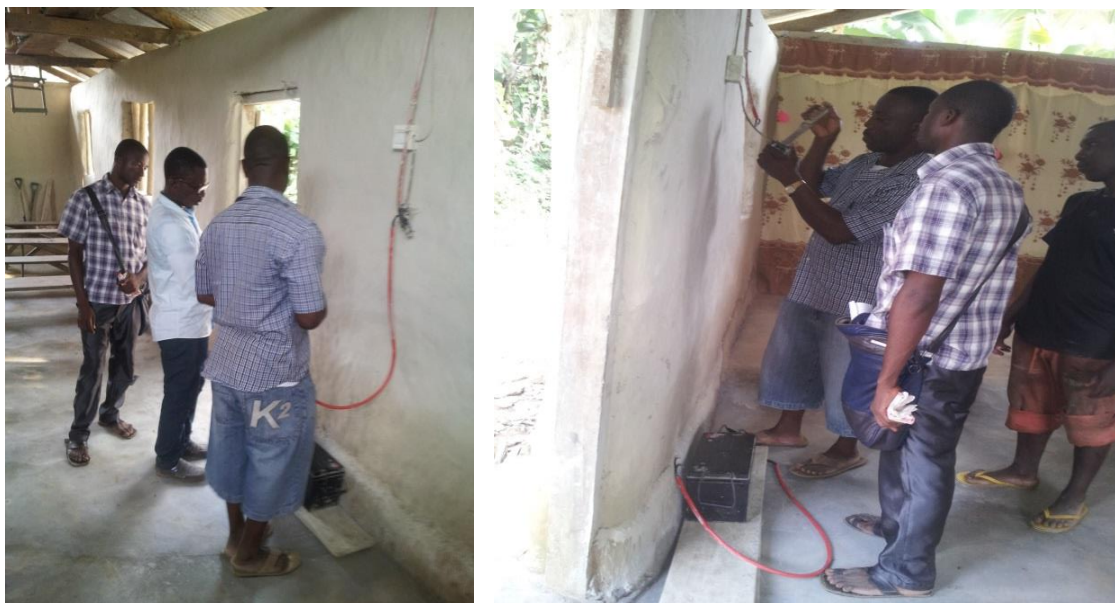
Figure 3-8 System components check at evaluation
