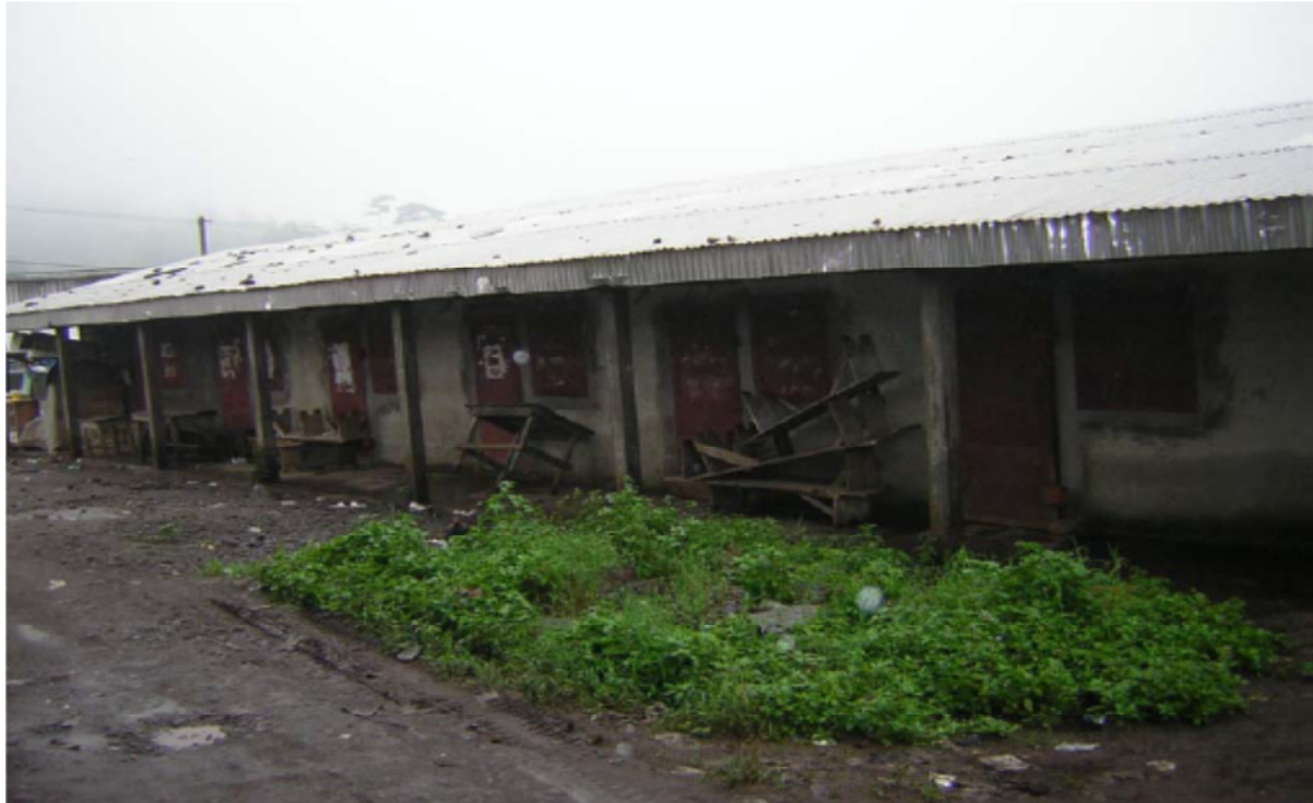
Figure 13: Corrugated iron sheets on a building in Buea.
