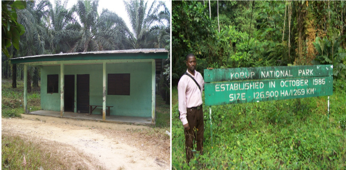
Figure 6. 2 Mana guard post and information board showing lack of maintenance
