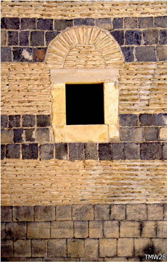
TMW28 Composite masonry combining stone ashlar with bricks in Byzantine architecture. Alternating brick and basalt masonry lines at Qasr Ibn Wardane, Syria, 564 AD.
