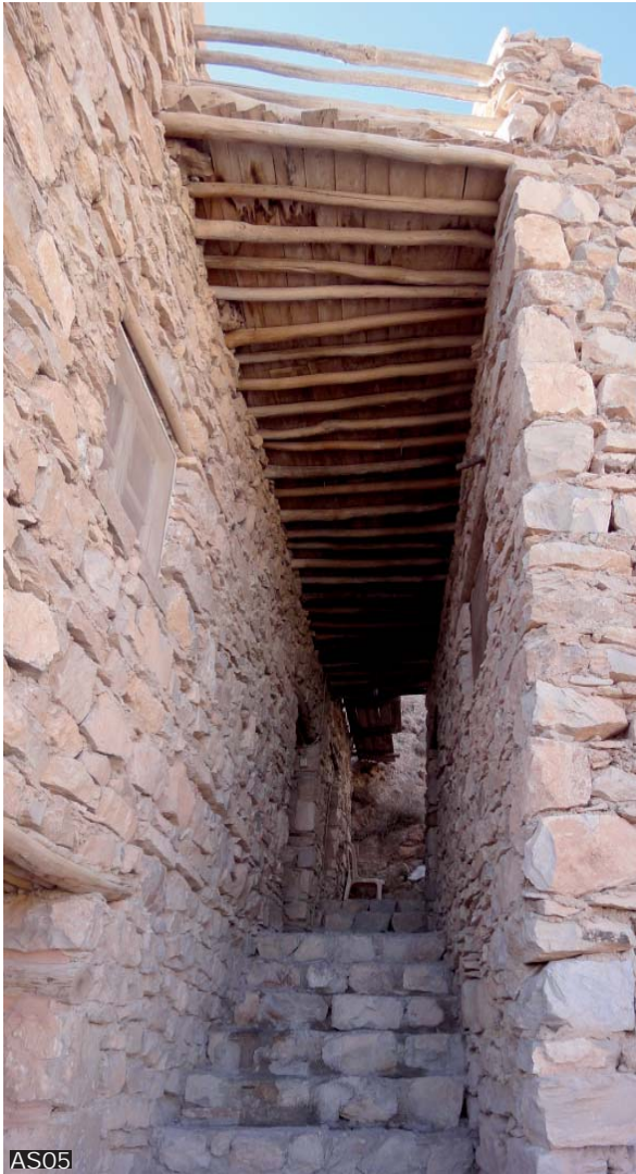
AS04-AS06 Utilization of locally available building materials and traditions combined with modern building techniques. For example, note a hidden load bearing structure of concrete at the Deir Al Huqab complimentary compound (photographs I. Helmedag).
