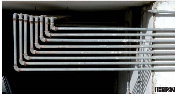
IH127 and 128 Supply and disposal pipes running along the façades of newly built apartment blocks. The lines could be better organized running in ducts.
