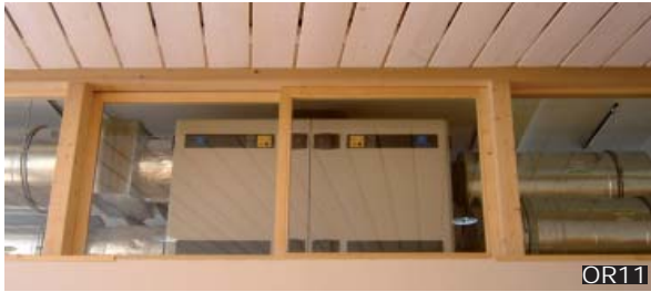
OR11 Ventilation as visible architectural component.
