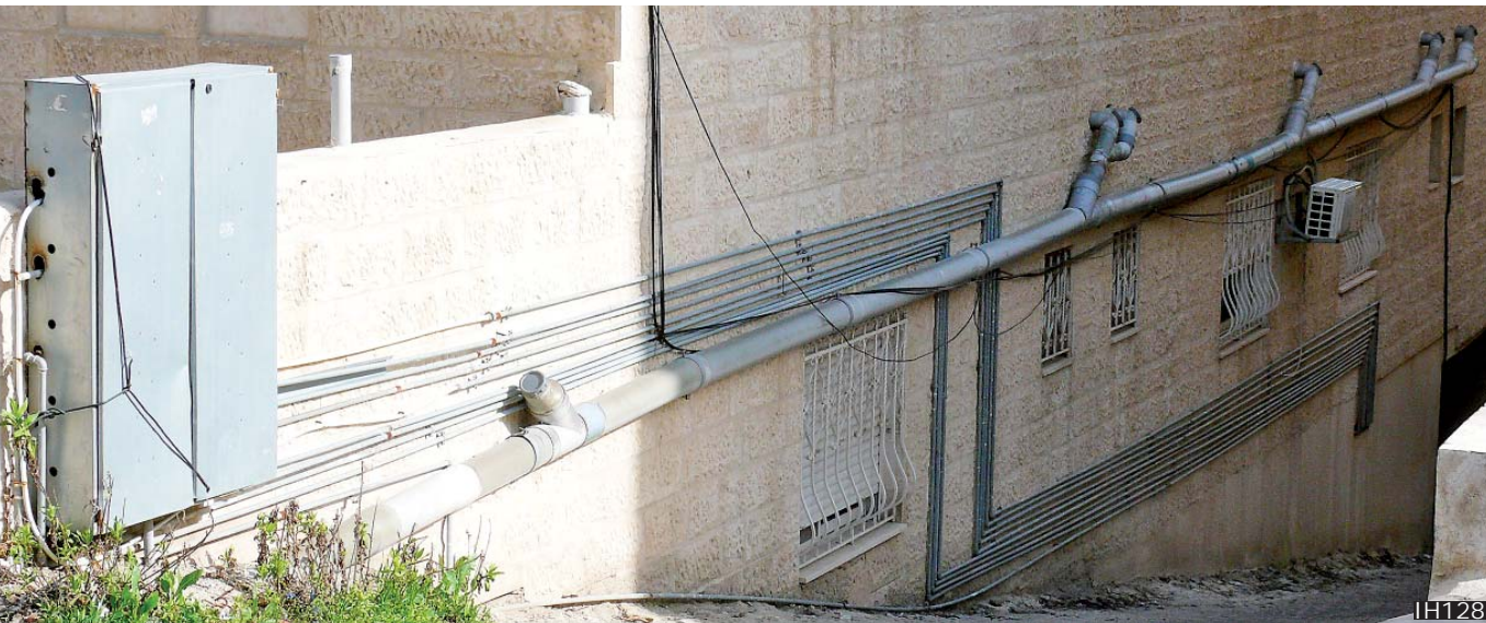
IH127 and 128 Supply and disposal pipes running along the façades of newly built apartment blocks. The lines could be better organized running in ducts.
