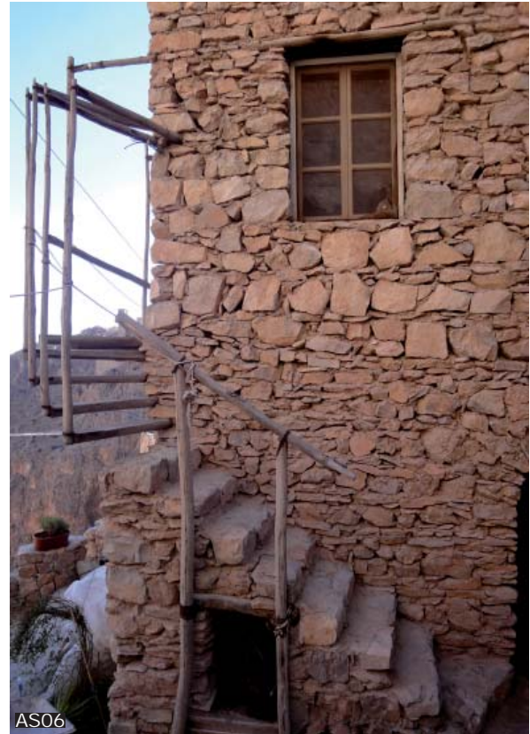
AS04-AS06 Utilization of locally available building materials and traditions combined with modern building techniques. For example, note a hidden load bearing structure of concrete at the Deir Al Huqab complimentary compound (photographs I. Helmedag).
