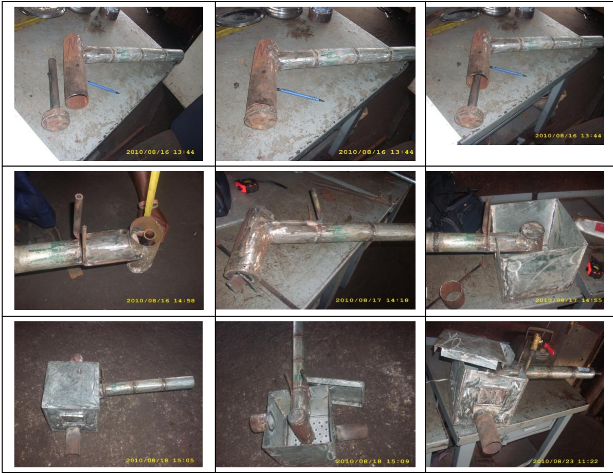
W: Construction of PG technology using 60-80% scrap metals
