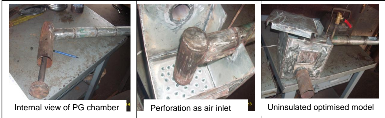
Figure 8.22 Construction of optimised PG technology in Lagos, Nigeria
