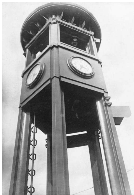
Figure 22: Traffic signal tower at Potsdamer Platz, Berlin, 1925. (Source: Bundesarchiv, Bild 102-01702)
