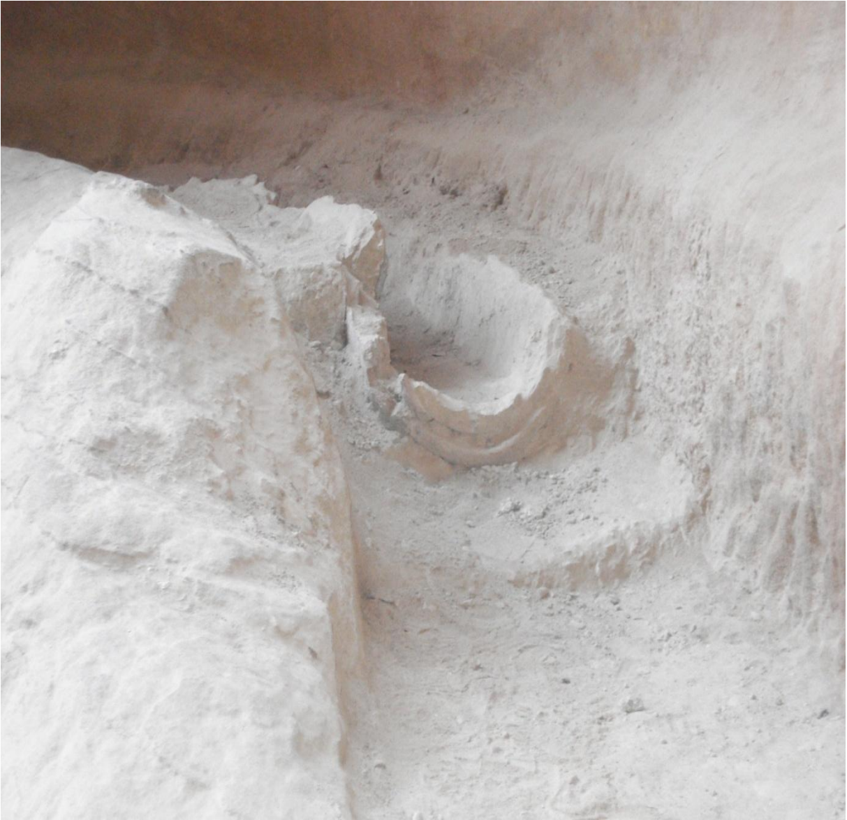
Figure 8: Hydraulic Pipe Remains
