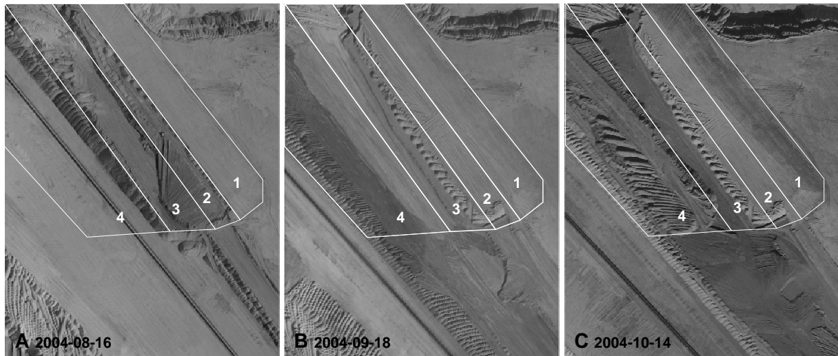
Fig. 10: Strip-wise construction north of the central clay dam can be clearly observed on aerial images (courtesy of Vattenfall Europe Mining AG, 2004).
