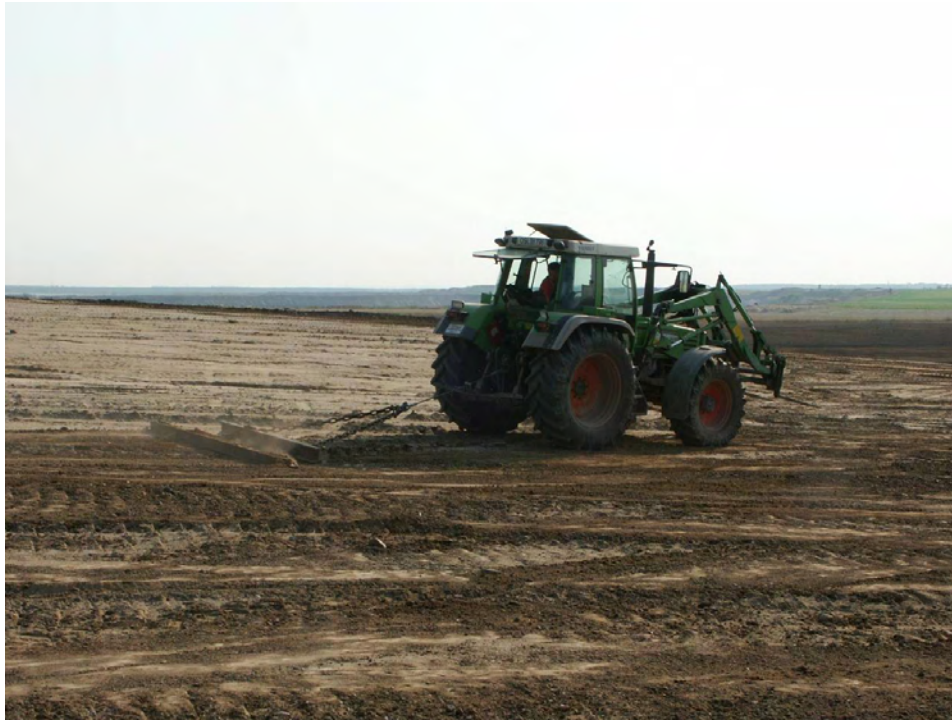
Fig. 16: Final flattening of the sandy surface and elimination of surface structures such as bulldozer tracks (September 2005).
