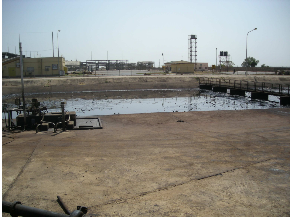
Figure 3.1 Waste Water Treatment Tank of NNPC Kaduna
