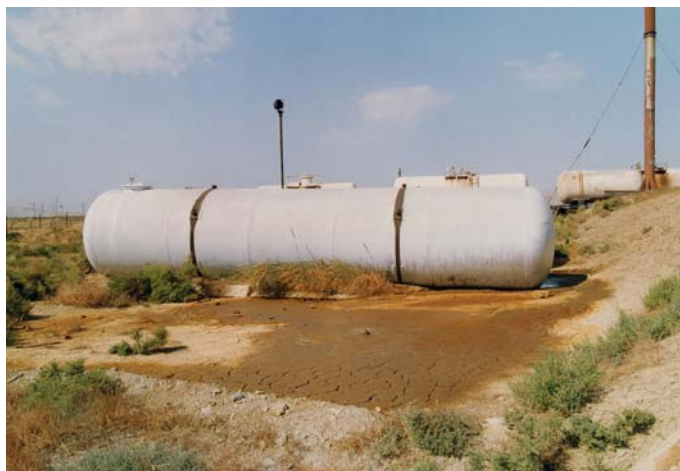
Figure 2-7: Leaking oxidizer (red fuming nitric acid) tank. Due to the leakage of the acid, soil iron has been oxidized – visible through red-brown coloring of the soil.
