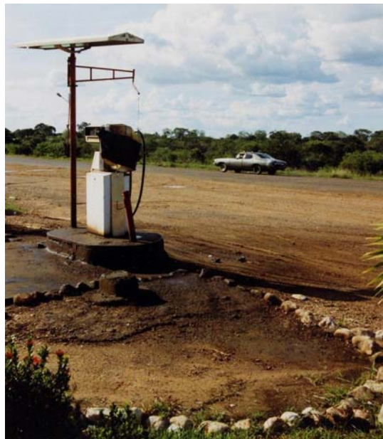
Figure 2-12: Photo of the small diesel filling station in the Rio Unare Basin in Venezuela, with clearly evident heavy diesel fuel contamination.
