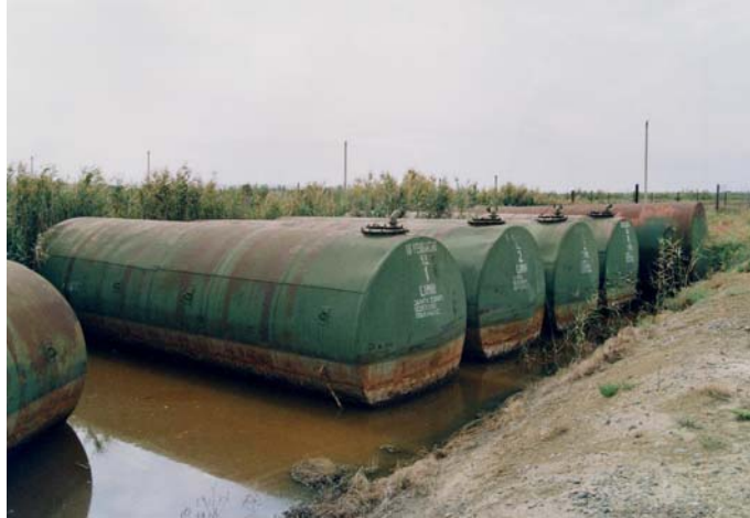
Figure 2-5: Steel storage tanks containing liquid rocket fuels (samine, kerosene, gasoline), stored in an open pit in contact with the groundwater. Fuels that leaked from the tanks are floating on the water.
