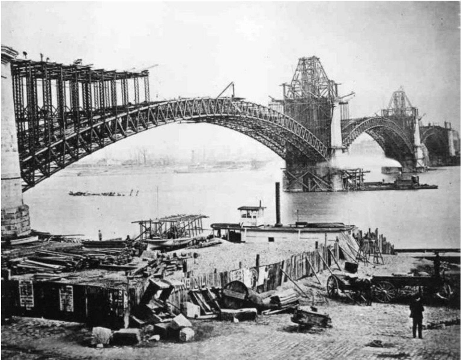
Construction of the Eads Bridge over the Mississippi in St. Louis (~ 1874)
