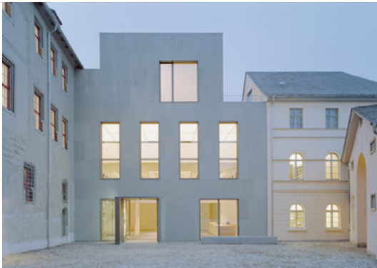
Fig. 4: The new entrance building set a new accent in the castle complex. © Klassik Stiftung Weimar. Ulrich Schwarz.
