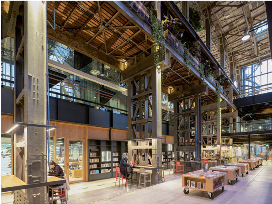
Fig. 1: The LocHal Library in a former locomotive shed. © Ossip Architectuurfotografie.
