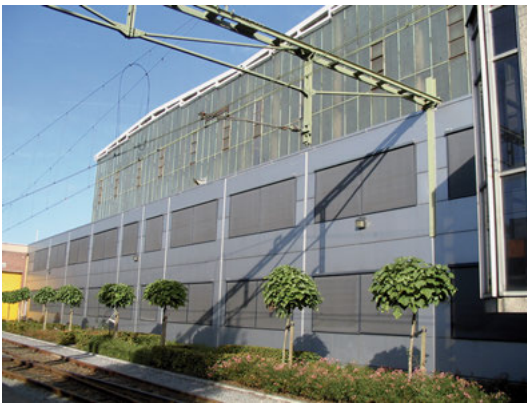
Fig. 2: The locomotive shed before restoration. © Rijksbouwmeester Atelier.
