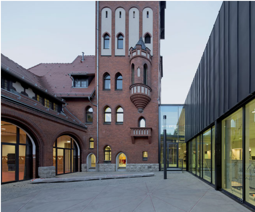
Fig. 10: The library's courtyard with the former hose drying tower and its false architectural elements used for fire brigade practice. © Werner Huthmacher.
