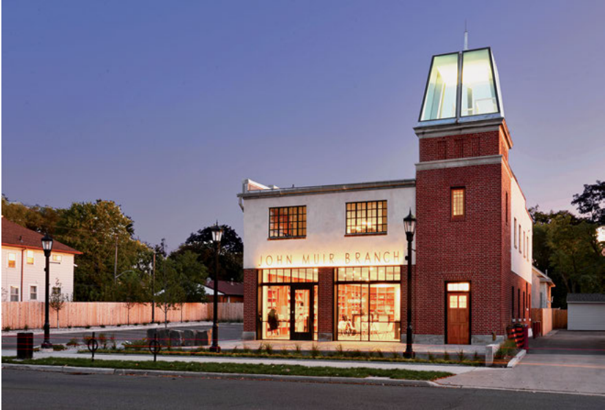
Fig. 1: Exterior of Windsor Public Library's John Muir Branch. © Jason Grossi, Studio g+G inc.
