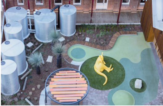
Fig. 9: Children's garden, water tanks. © Brett Boardman.
