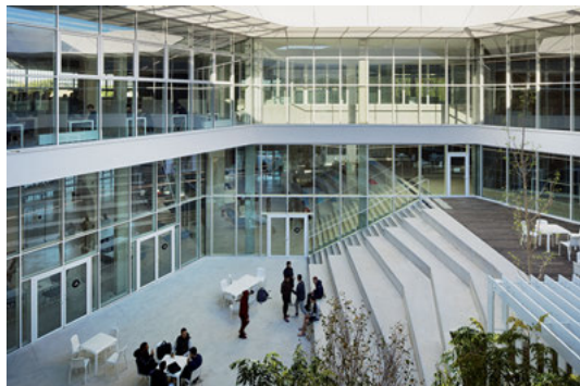
Fig. 7: The patio. © Takuji Shimmura.
