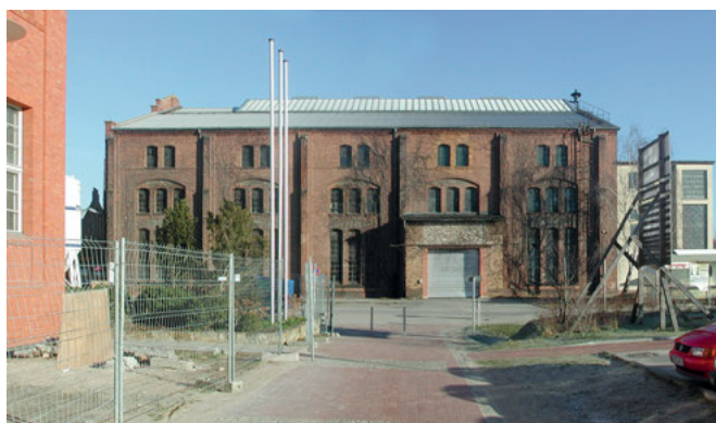
Fig. 2: The exterior of Hall 10 in 2002. © Robert Niess.
