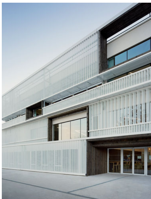
Fig. 12: Front detail view. © Takuji Shimmura.
