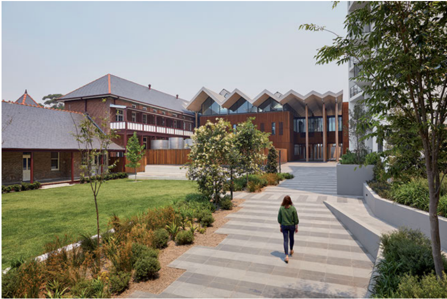
Fig. 8: Northern view from Hospital Lane. © Tom Roe.
