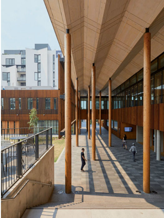
Fig. 4: Reinstated Hospital Lane. © Brett Boardman.
