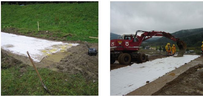
Figure 7.10: The geotextiles with applied optical cables in Solina ( left ) and Swinna Poremba ( right ).
