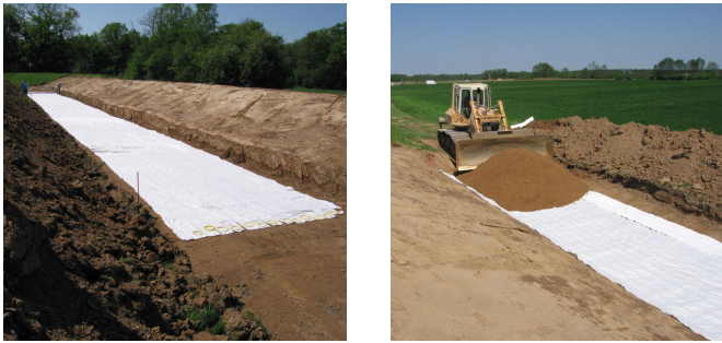
Figure 7.8: Photographs from the construction site in Dessau-Sollnitz during the first attempt to integrate sensor-equipped geosynthetics into the soil body of a river dike.
