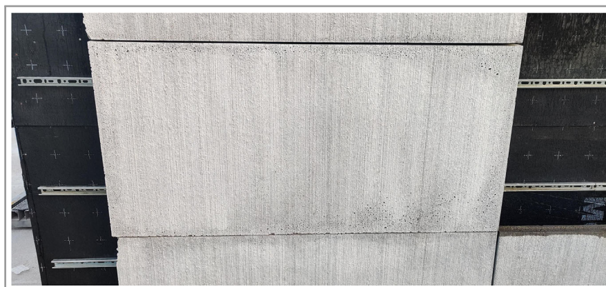
Figure 4. Facade element made with infra-lightweight concrete manufactured by Beton und Naturstein Babelsberg GmbH.
