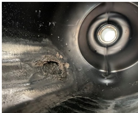
Fig. 4. Internal view of the damaged pressure vessel.
