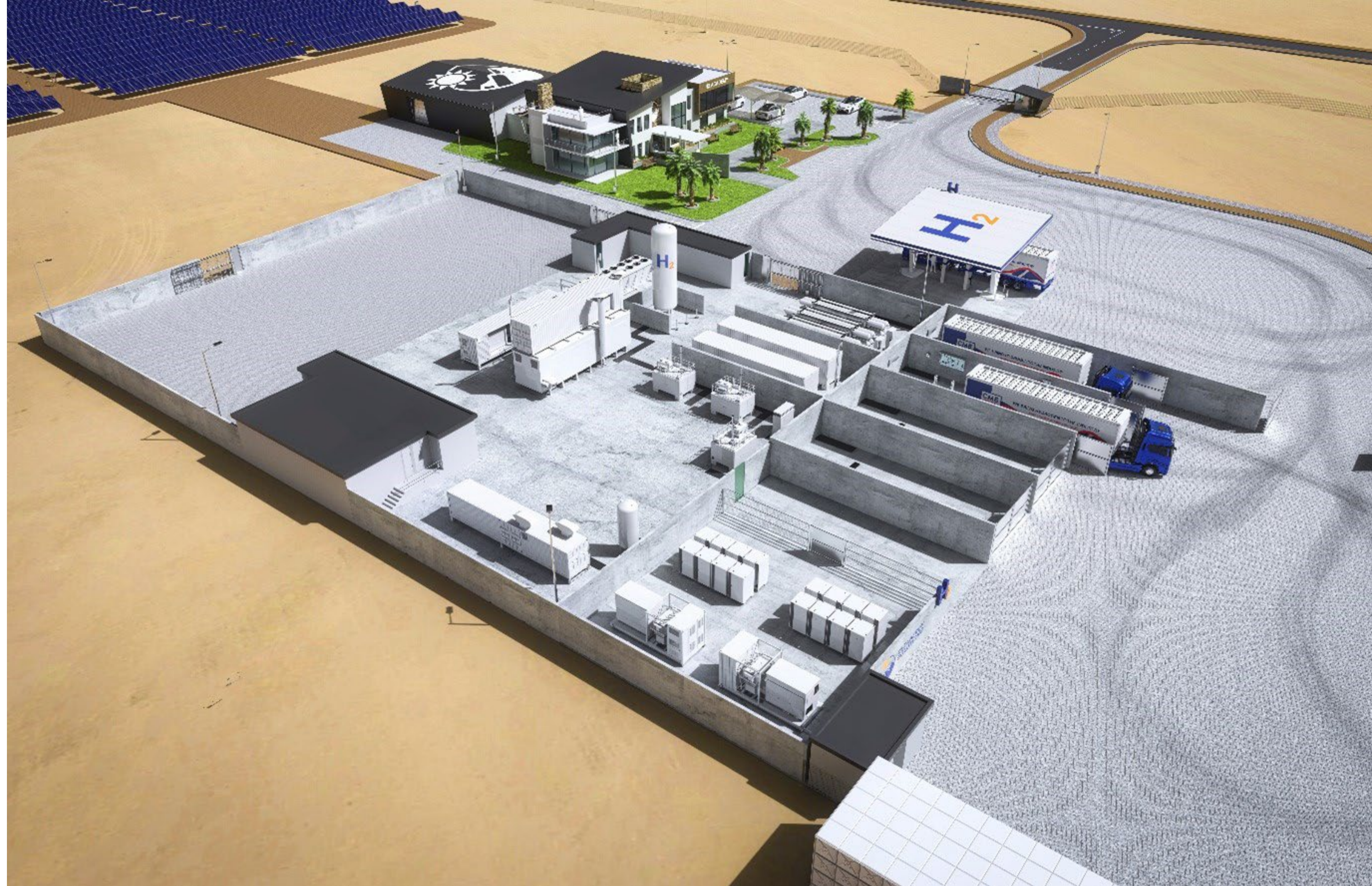
A pilot plant for the production of green hydrogen is being built near Walvis Bay, Namibia.
