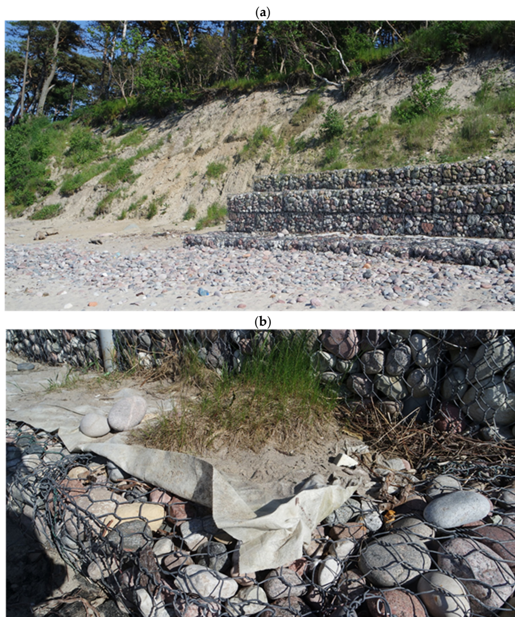
Figure 1. Geotextiles used as cover for gabions in coastal protection. Location: Swetlogorsk, Oblast Kaliningrad, Russian Federation (a) total view, (b) detail view with uncovered geotextile.
