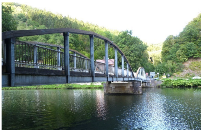
FIGURE 1 Measurement object “Lenne Bridge” made of galvanized steel over the Lenne river on the German federal highway B236. [Color figure can be viewed at wileyonlinelibrary.com ]
