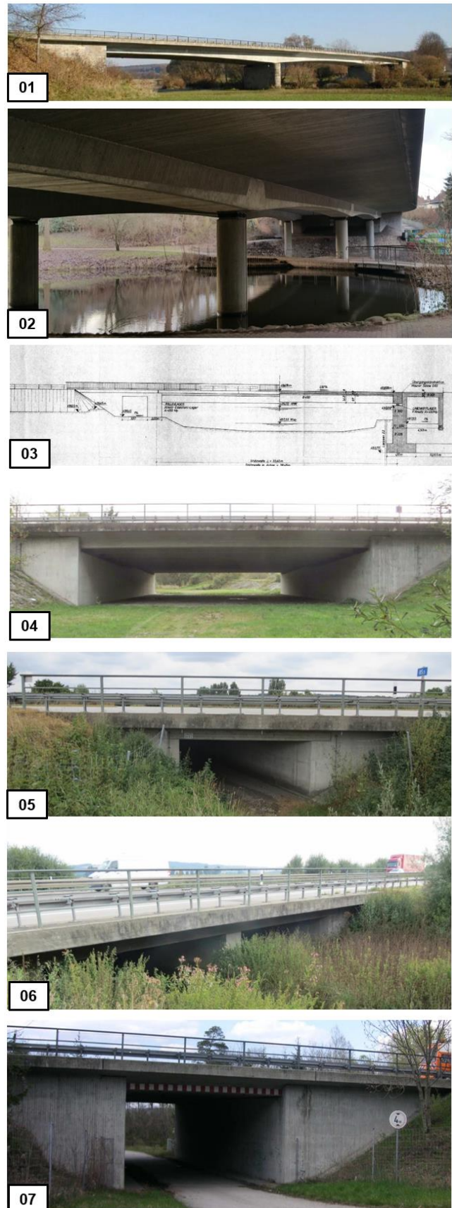
Figure 3 Overview of the selected bridges
