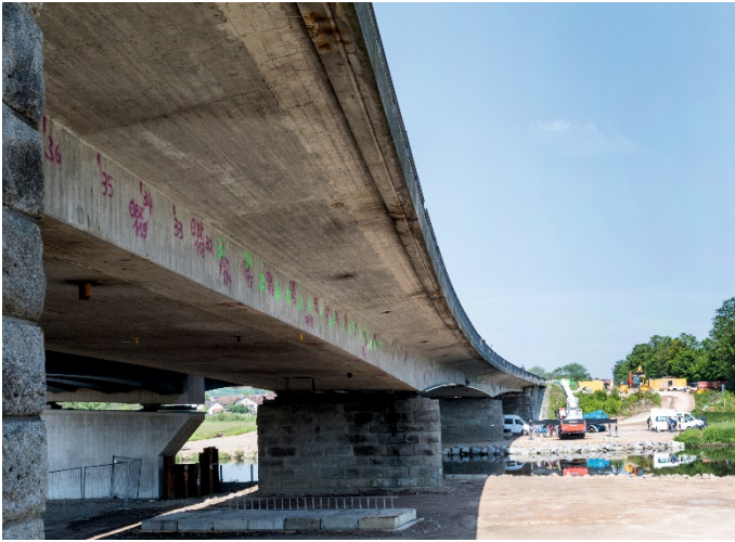
Figure 2. The investigated prestressed concrete bridge.
