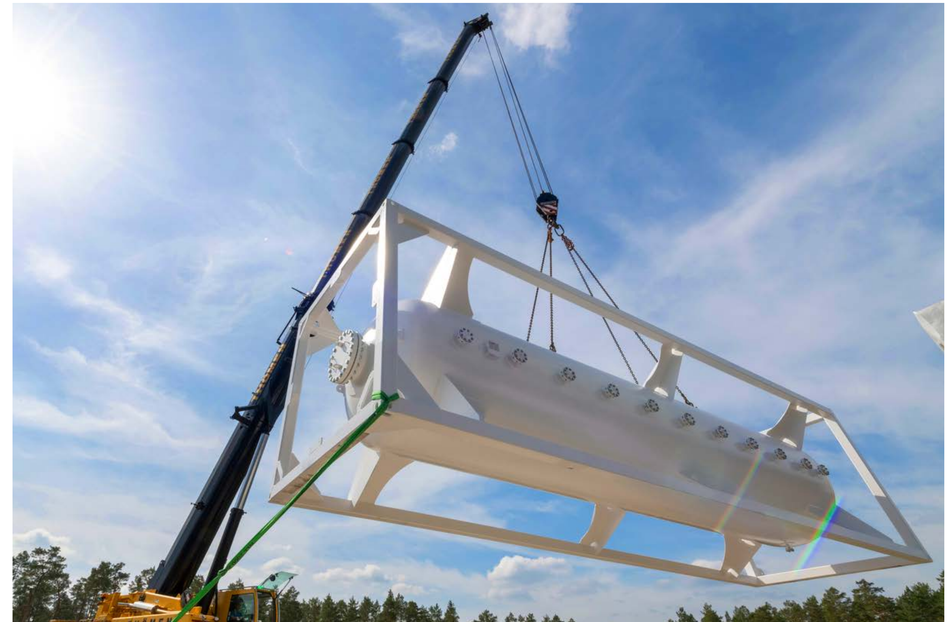
A special crane delivers the 60-cubic-metre tank
