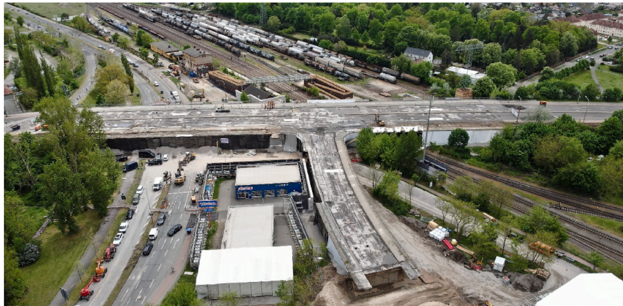
Fig. 2. Aerial photo of the “Altstadtbrücke Brandenburg” shortly before it was blasted. Viewer looks south.
