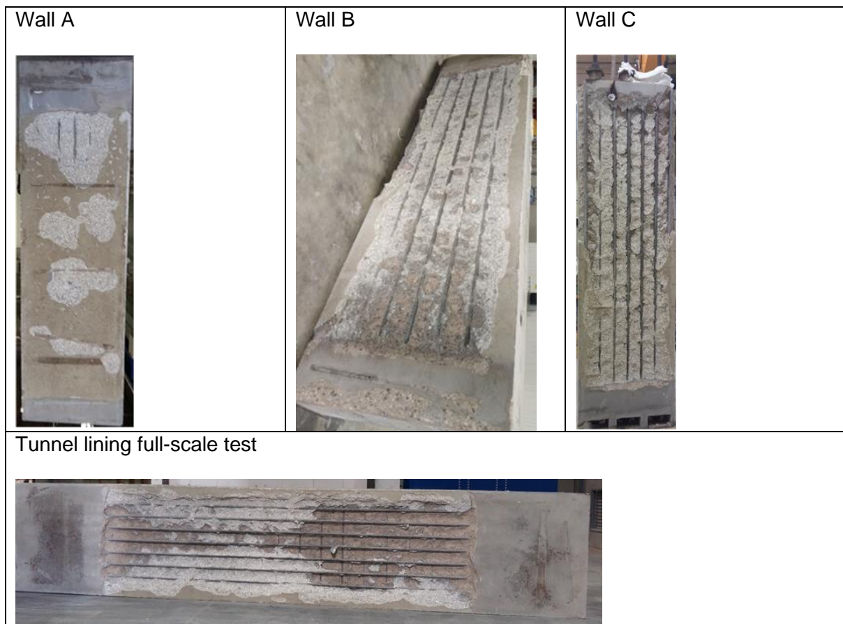
Figure 3 Exposed face of the walls and tunnel lining full-scale test at the end of the fire tests for the CETU research program
