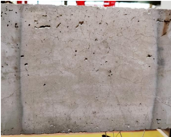
Figure 11 the exposed face of the sample after exposure to simulated ISO 834 fire curve
