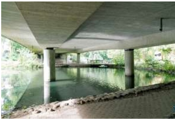
Fig. 4. Photo of the investigated prestressed concrete bridge
