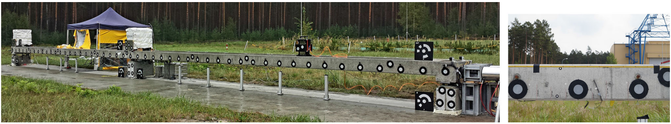
Fig. 12 Bridge example: Two span concrete test bridge at BAM testing side (left) and occurred crack pattern in the middle of the first field (right)
