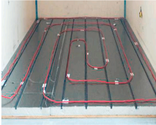
(a) pipeline arrangement
