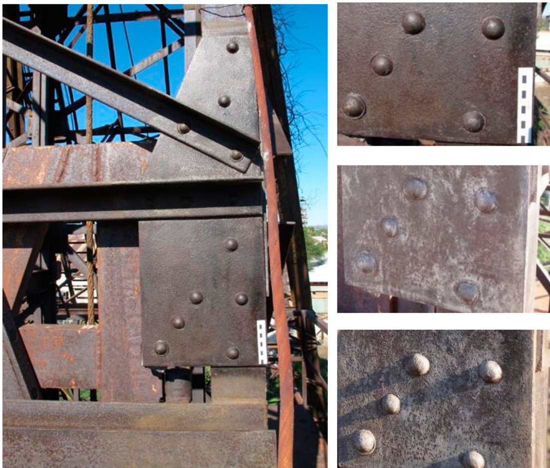
Figure 5. Samples of Tecero® Wax coating. The right images show the condition on May 2018 (top), November 2018 (middle), and October 2019 (below), respectively.
