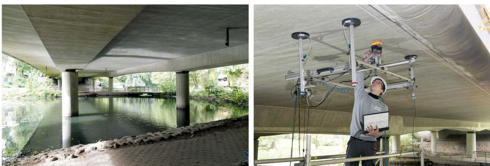
FIGURE 1 Photos of the investigated bridge (left) and of the mounted structure scanner equipped with a GPR antenna (right; extracted from (Maack, Küttenbaum, Epple, & Aligholizadeh, 2021) 8 )
