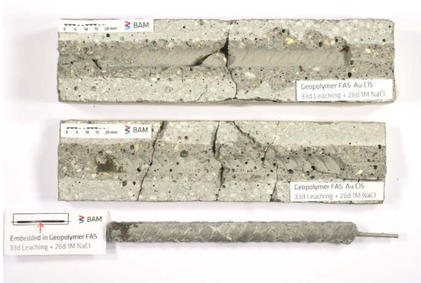
Figure S15. Mortar specimen FA-L-Cl 5 and embedded steel rebar split after depassivation of the steel was detected.
