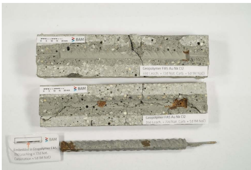
Figure S18. Mortar specimen FA-L-A-Cl 2 and embedded steel rebar split after depassivation of the steel was detected.
