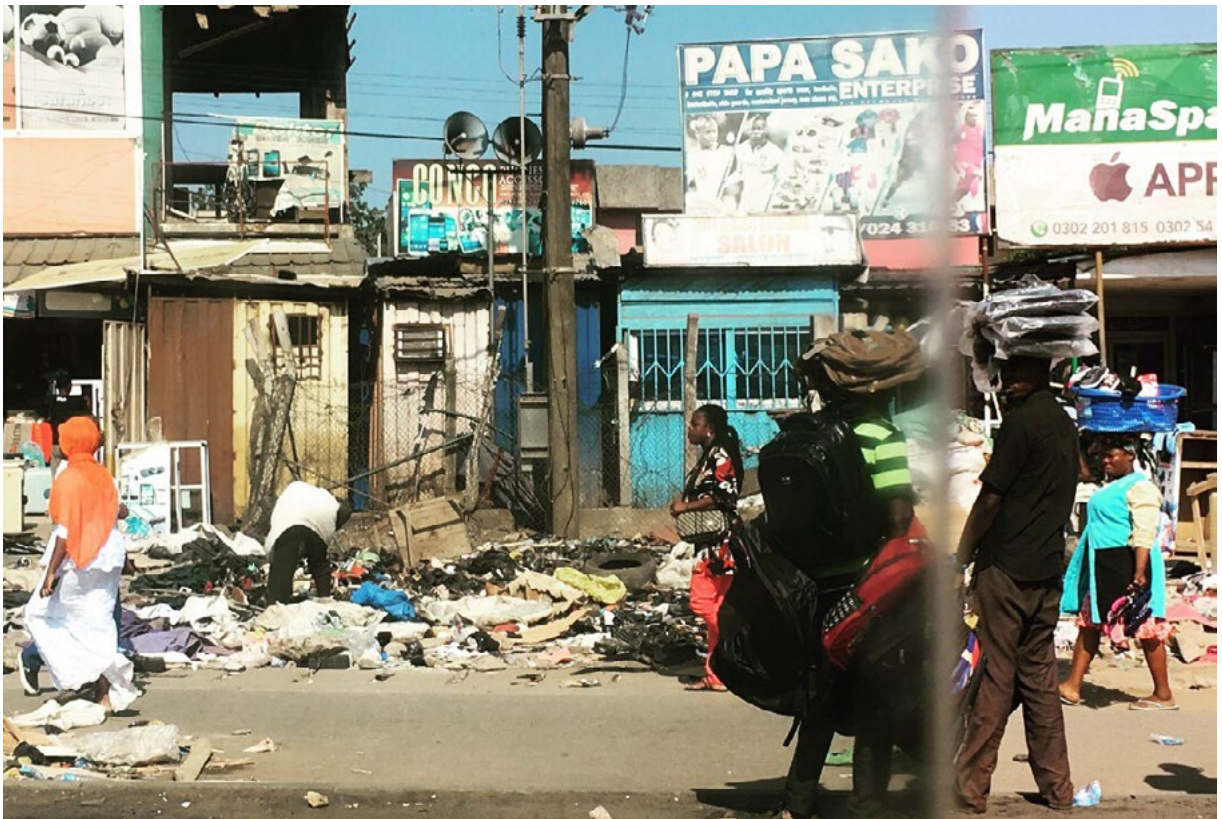
The aftermath of vendor stall demolitions at Madina Zongo Junction, Accra, July 2018. N. Serumaga-Musisi, 2018
