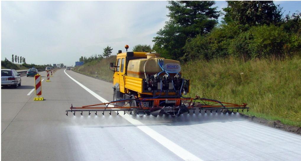
*and distribution of additives. Up to now this has prevented widespread practical application of the technically and highly efficient deep hydrophobisation because the risks of failure are too high without a suitable quality control to match the usual building process.*
