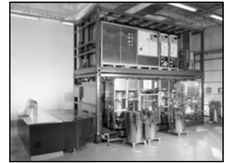
Containerized modular plant Source: INVITE GmbH
