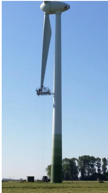
Fig. 2: stopped wind turbine during maintenance inspection using a special platform
