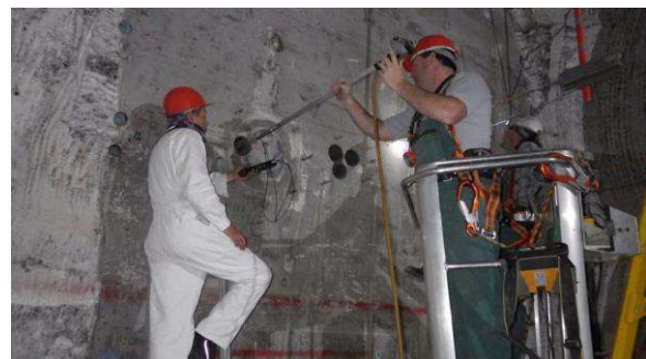
Figure 3. Borehole probe applied at the sealing construction
