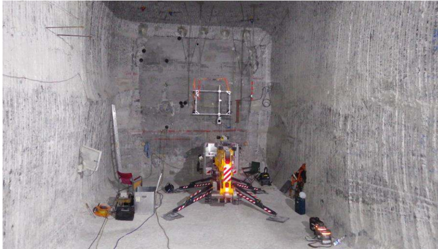
Figure 1. Front side of the sealing construction during experiments
