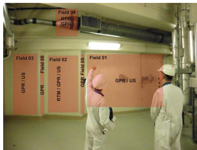
Figure 1: Overview of measuring areas for non-destructive testing at the outer side of the containment [1][3]
