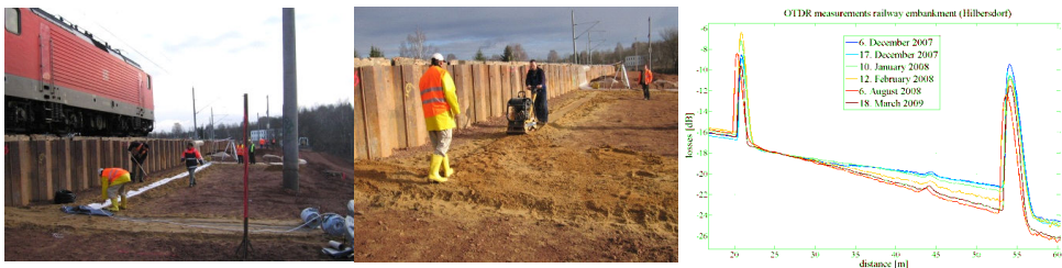
Figure 12. Installation of POF-equipped geotextiles in a railway embankment near Chemnitz, Germany (left and middle) and OTDR traces measured on the textile-integrated POF (right).
