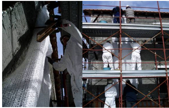
Figure 20. Application of technical textiles containing POF on a masonry building at the Eucentre in Pavia, Italy.
