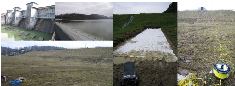
Figure 6. Gravity dam in Solina, Poland (left) and the construction site with the sensor-based non-woven geotextile before embedding in the soil and 3 years later (right).
