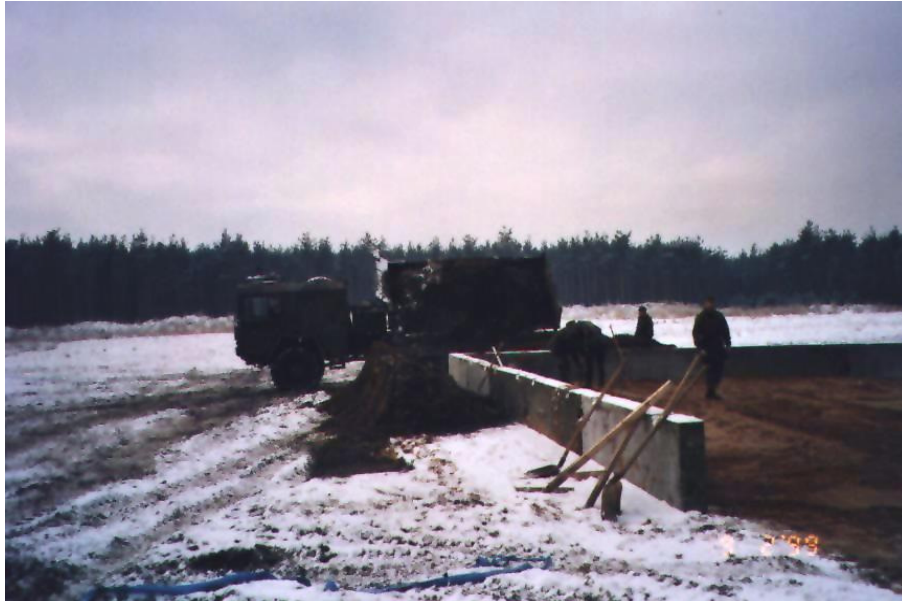
Fig 5.1: Setting up the external sidewalls
