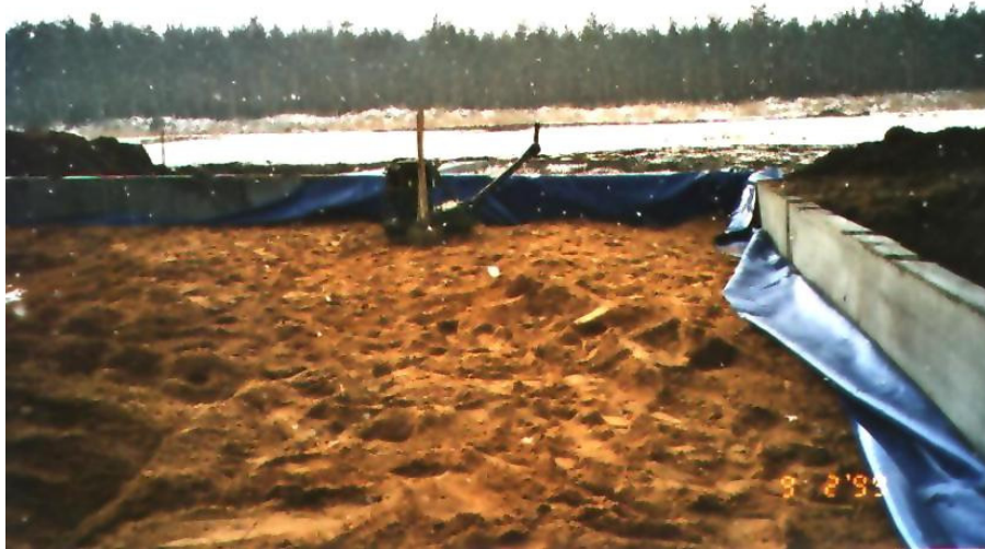
Fig. 5.4: Applying the layer of gravel
