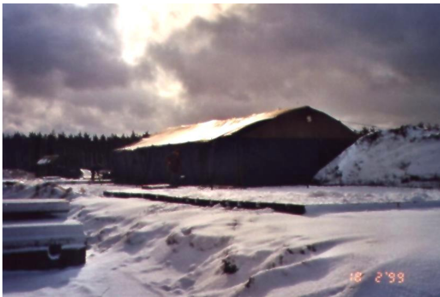
Fig 5.8: The welding site for the fire trough for the RTC
