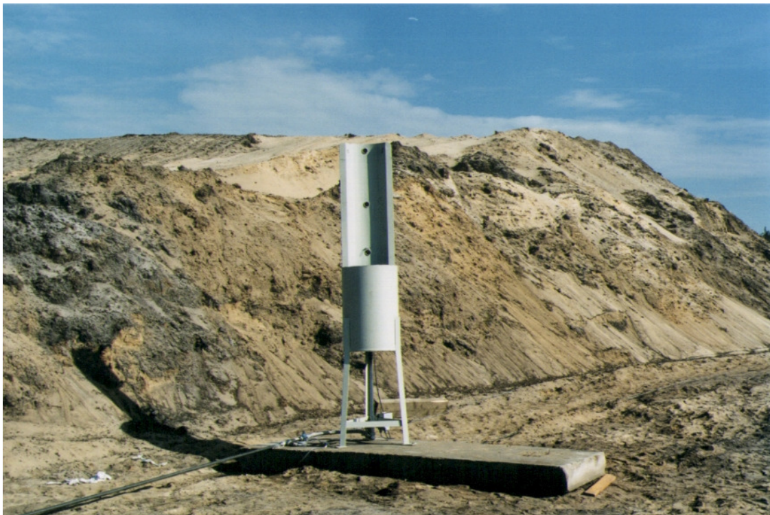
Fig. 6: Relief facility outside the protective embankment
