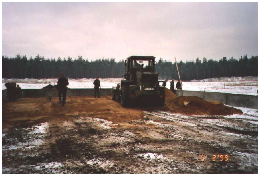
Fig. 5.2: The first layer of gravel is installed
