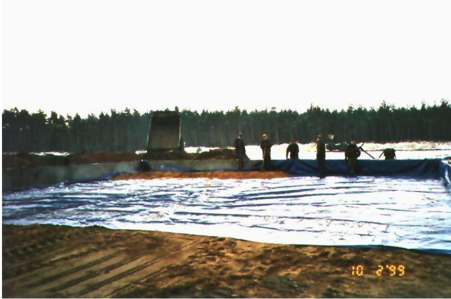
Fig. 5.3: Installing the oil-resistant sheet
