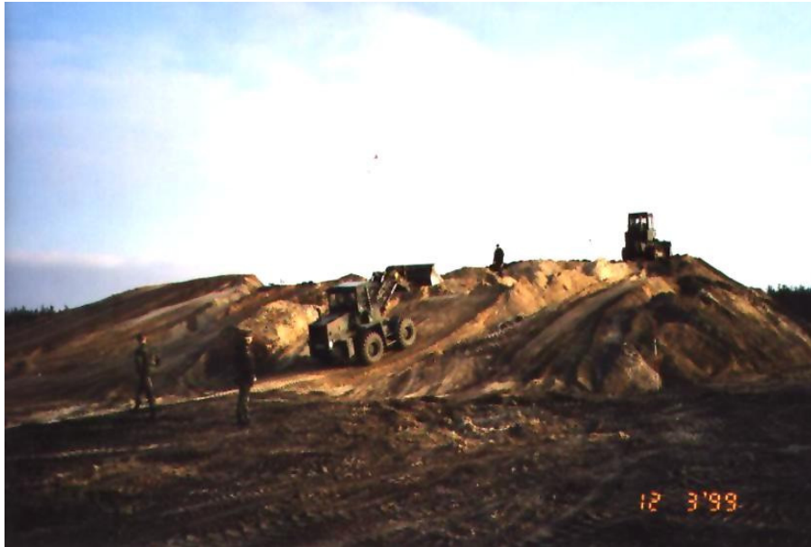
Fig 5.7: Building the earth embankment for the fire stand.
