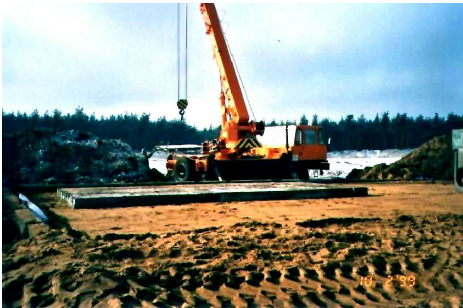
Fig 5.6: Laying down the cover slabs
