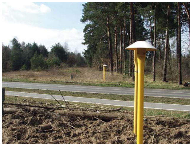
Figure 1: Route marking of a natural gas pipeline passing under a road.
