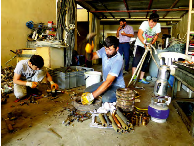
Figure 5.11: Dismantling elevator parts 15
