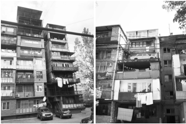
Figure 7.10: Building extensions: kamikaze loggias and rooftops additions in Gldani
