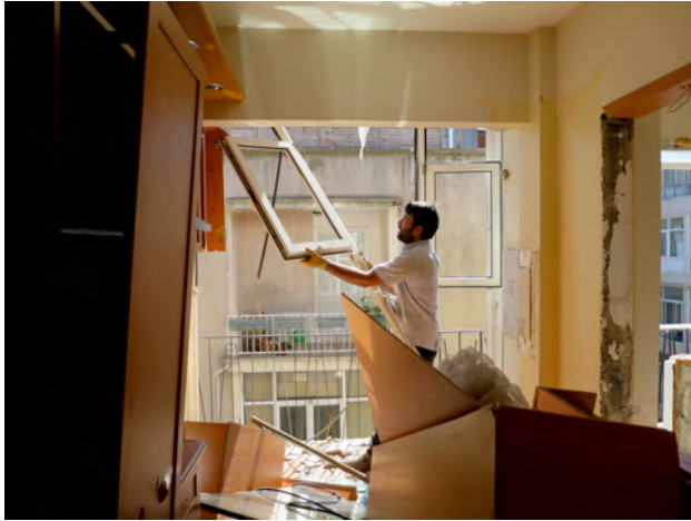
Figure 5.8: Dismantling PVC frames 11
