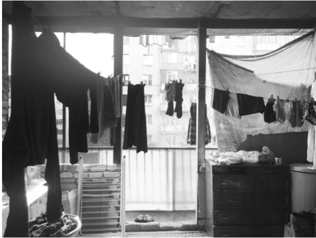
Figure 7.11: Unfinished facade in Gldani
