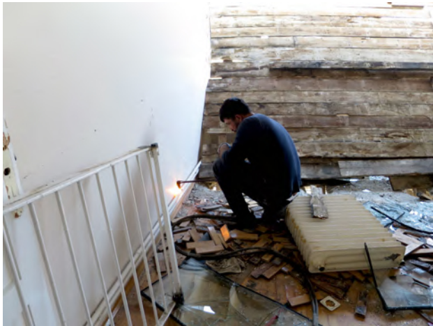
Figure 5.7: Cutting metal pipes 10
