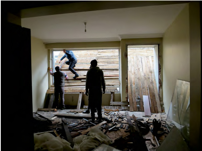
Figure 5.6: Installing the debris slide 9
